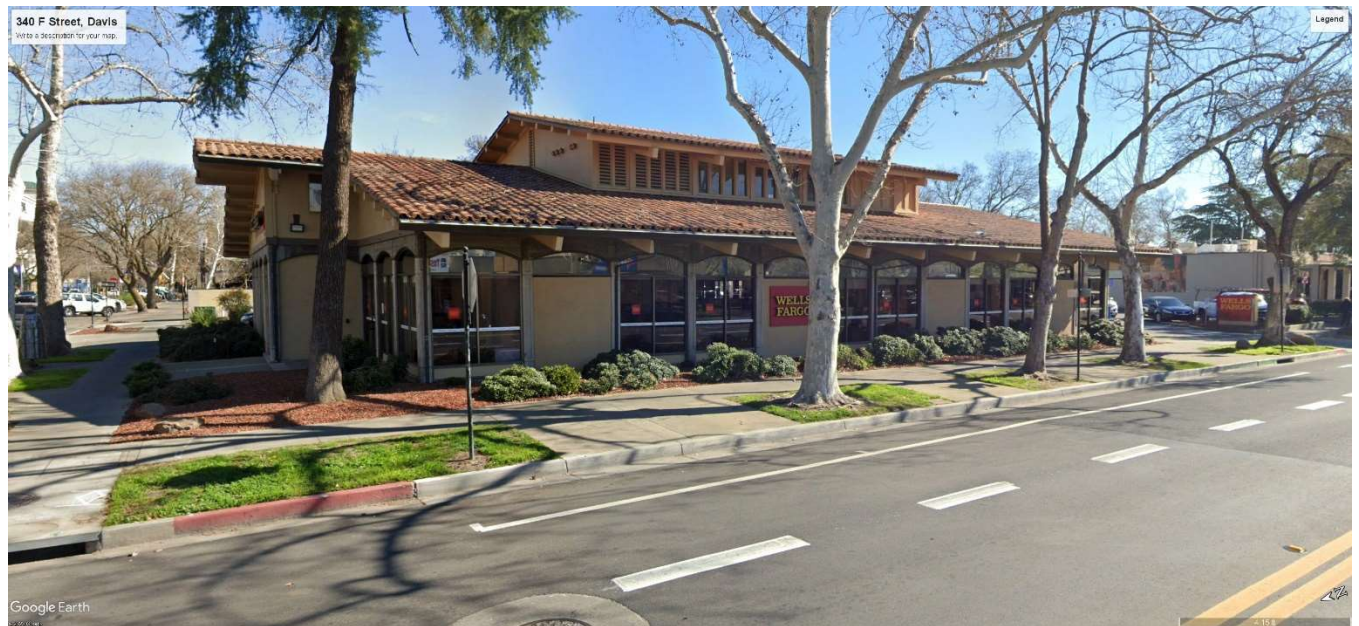
Figure 2 – 340 F Street Front view (Google Earth 05/03/2023)
